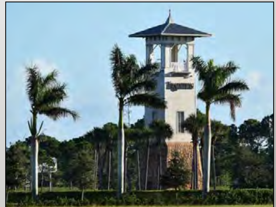
Figure 53 The Tradition DRI has employed a signature tower design to brand the community. Credit: TCPalm
