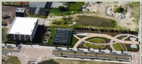
A central utility plant provides stormwater and cooling services for the entire Tampa Housing Authority's Encore! development. At right is the underground stormwater vault, capped by a park and solar panels. At left is the central chiller plant, which can efficiently cool up to 2.5 million square feet of space. These utility decisions enable a more resilient community.
