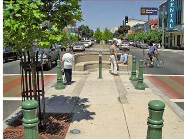
Pedestrian Median w/ Bollards & Street Furniture
