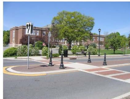
Pedestrian Refuge Island / Enhanced Crosswalk w/ Bollards
