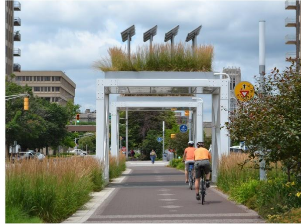
Architectural Feature w/ Green Roof
