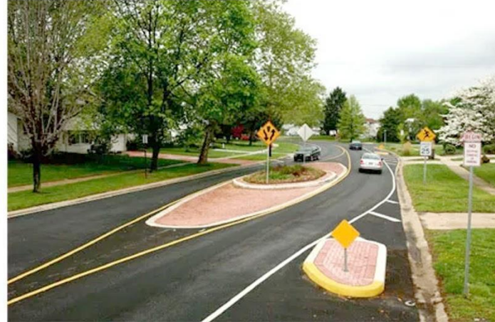
Center Median Island / Chicane
