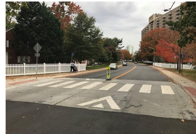
Raised Pedestrian Crossing
