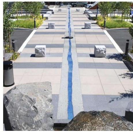
Enhanced Crosswalk w/ Textured Pavement & Street Furniture
