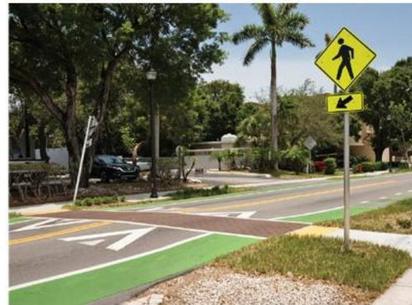
Raised Textured Ped Crossing / Speed Hump
