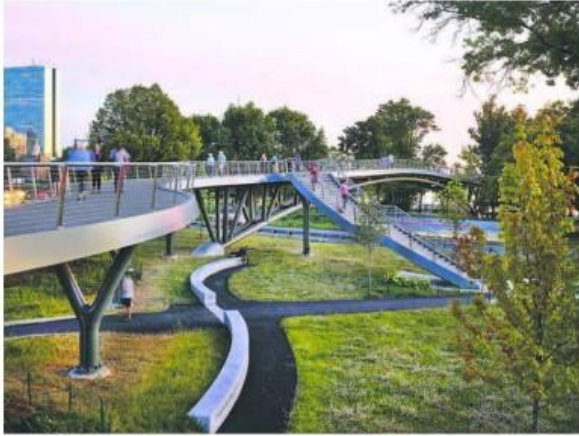
Raised Walking Path / Bridge
