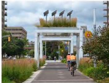
IMAGE 2: UNDERPASS STRUCTURE WITH GREEN ROOF
