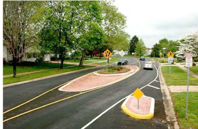
Center Median Island / Chicane
