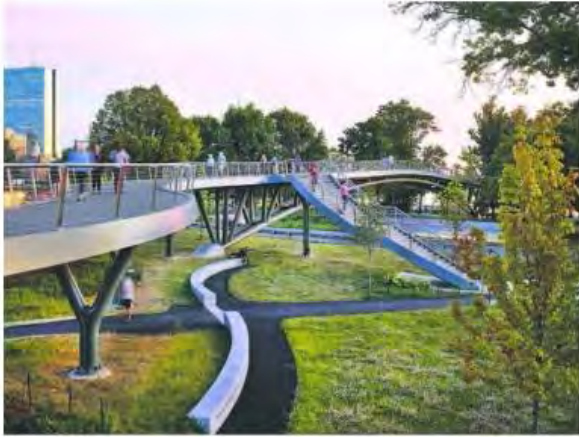
Raised Walking Path / Bridge
