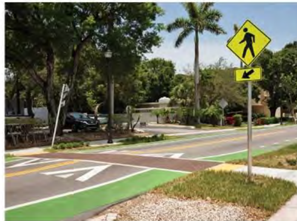
Raised Textured Ped Crossing / Speed Hump
