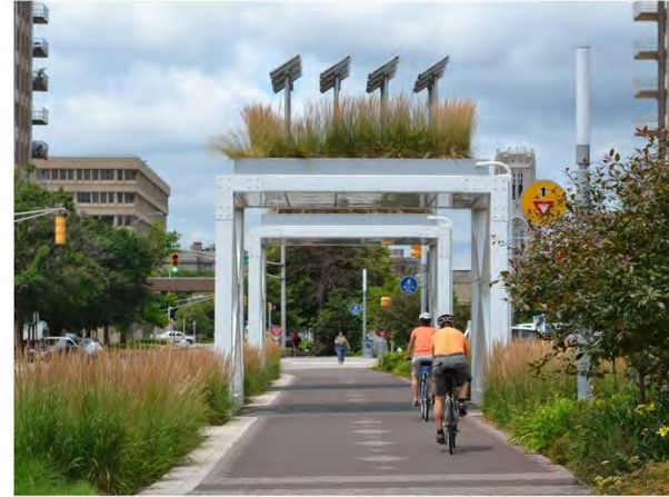
Architectural Feature w/ Green Roof
