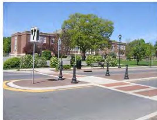
Pedestrian Refuge Island / Enhanced Crosswalk w/ Bollards
