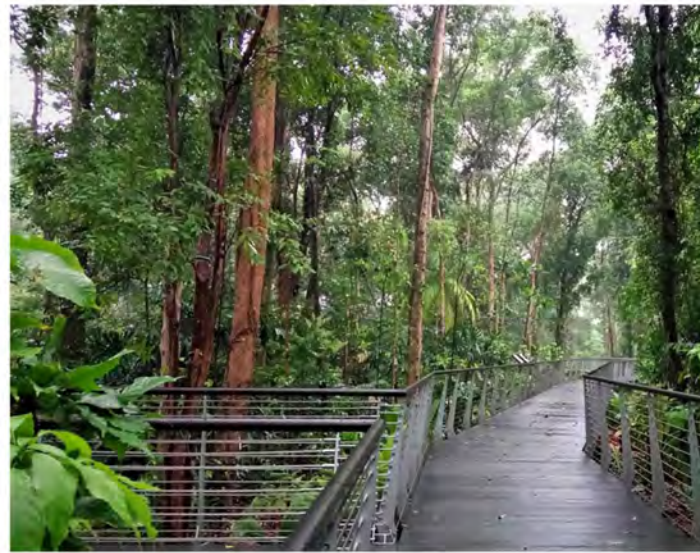
IMAGE 2: ENCLOSED BOARDWALK- METAL
