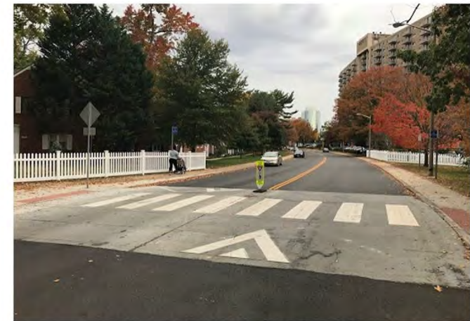
Raised Pedestrian Crossing
