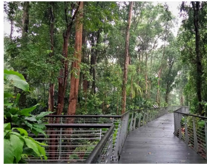
IMAGE 2: ENCLOSED BOARDWALK- METAL
