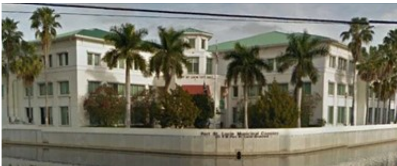
Figure 3-2: Florida Vernacular Architectural Style
