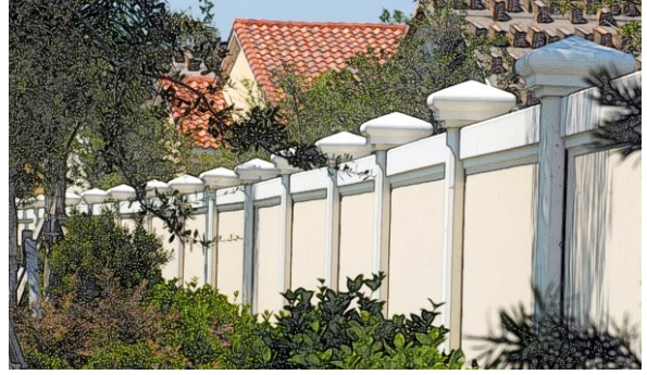
4 Masonry wall buffering
