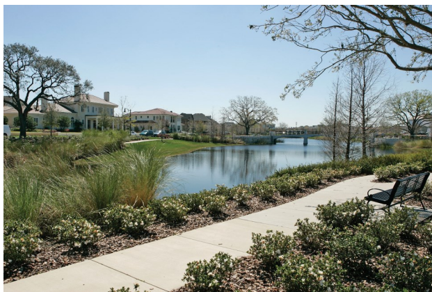
Stormwater park (Source: Skip Milos Productions)
