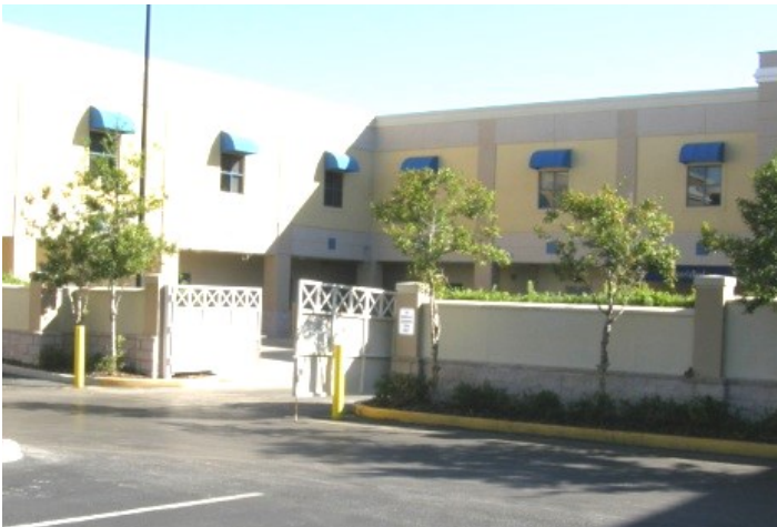
Service area screening
