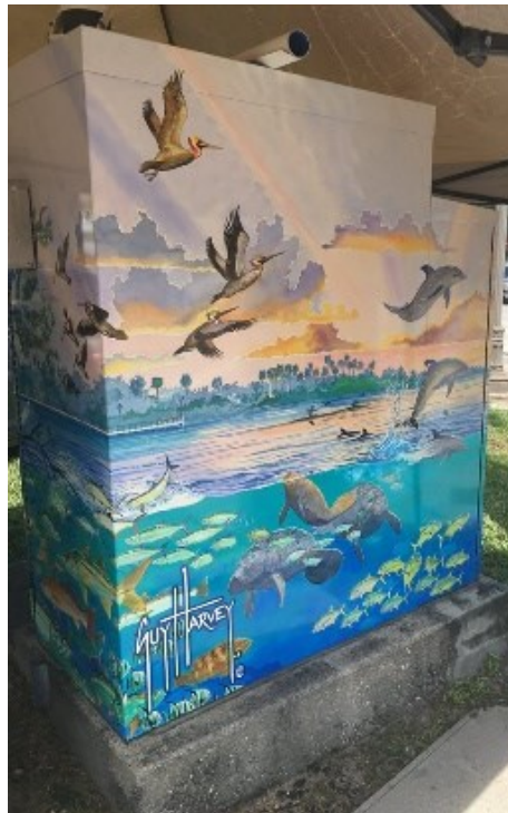
Signal Box Wrap (Source: City of Port St. Lucie, FL)
