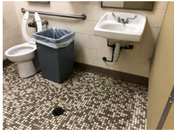
Photo: Flush Valve Water Closet
