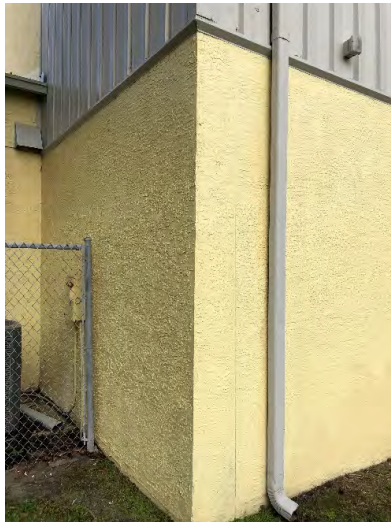
Photo 4.5: Typical building corner
