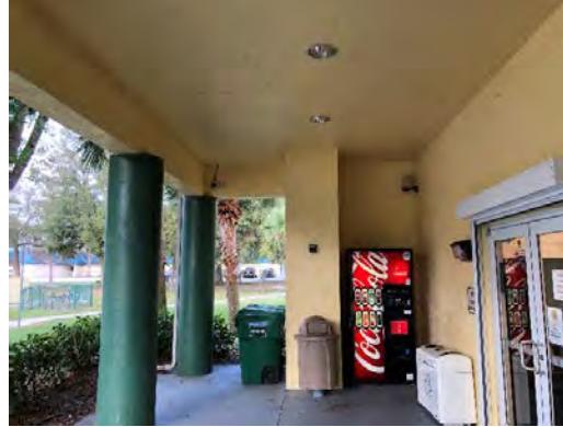
Photo 3.6: Concrete beam and columns at the front entrance
