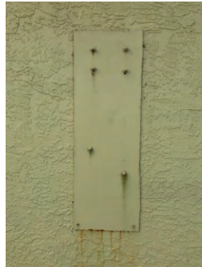
Photo 4.6: Steel plate bolted to the exterior face of the back CMU
