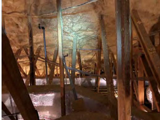
Photo 6.7: Clubhouse wood roof trusses, roof insulation and sprinklers
