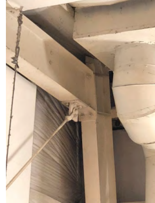
Photo 5.6: Lateral X-Bracing top connection to the building frames
