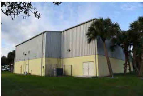
Photo 7.13: exterior metal wall panels.
