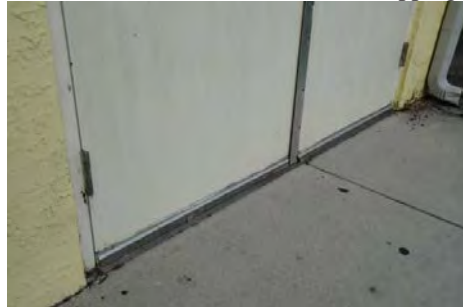
Photo 8.2: Exterior door weather stripping.
