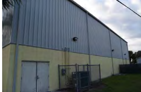
Photo 7.12: Exterior metal wall panels.
