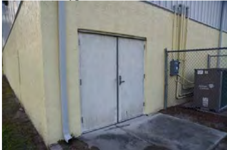
Photo 8.1: Typical exterior door condition.
