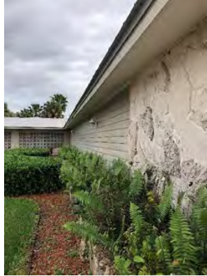
Photo 4.9: Masonry planter walls along the exterior load bearing masonry building wall
