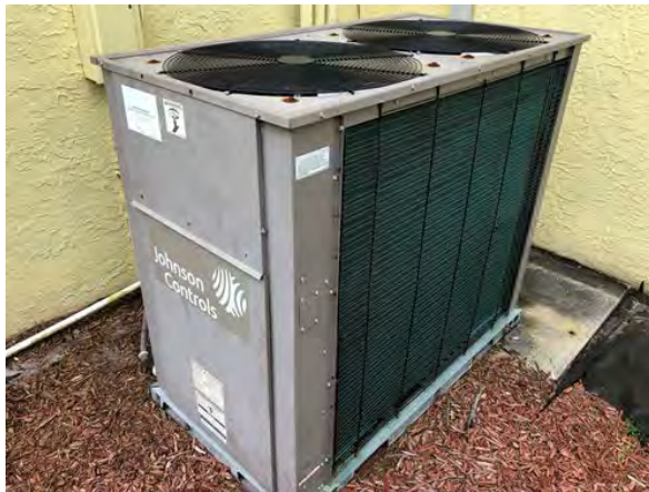
Photo: Gymnasium NE
