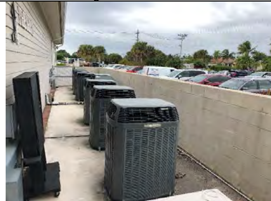
Photo 3.2: Concrete slab on grade at the open mechanical equipment enclosure along the front entrance building elevation
