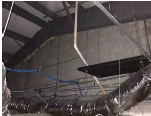
Photo 4.1: masonry wall at the low entrance roof
