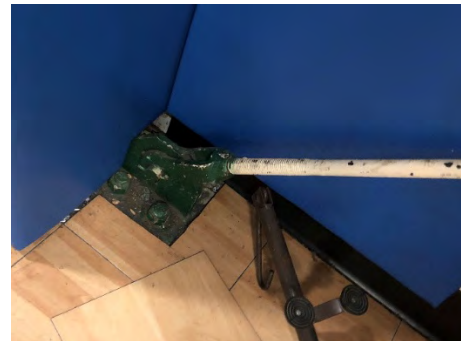
Photo 5.4: Lateral X-Bracing bottom connection
