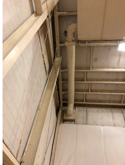
Photo: Gymnasium SW AHU – O/A Intake
