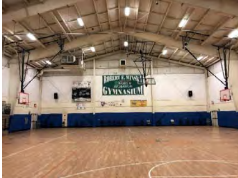
Photo 5.13: Overall roof framing view
