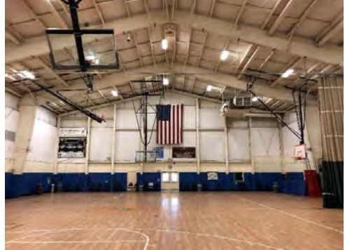
Photo 5.14: Overall roof framing view
