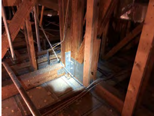
Photo 6.5: Clubhouse wood roof trusses connections
