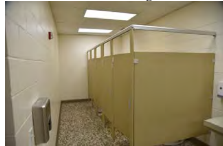
Photo 9.2: Bathroom tile in good condition.
