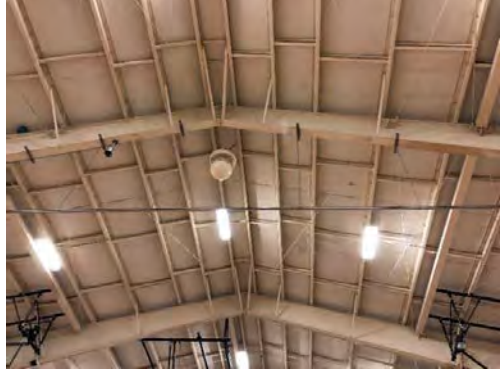
Photo 5.12: Moment frames, roof purlins and hanging partition wall support framing
