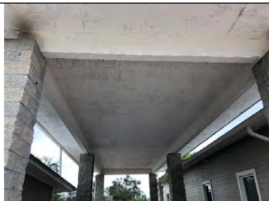
Photo 6.14: Walkway canopy ceiling finish
