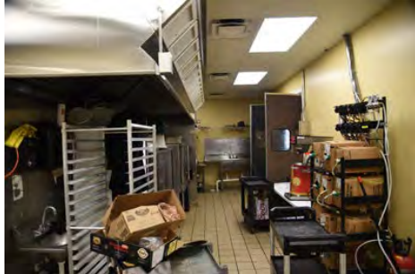
Photo 8.7: Specialty double swing doors at the kitchen.
