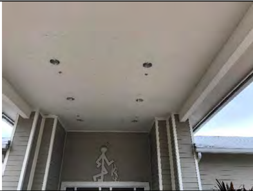
Photo 5.3: Steel beams with some surface rust at the front entrance port cochere
