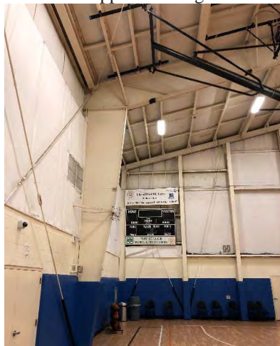
Photo 5.15: Basketball board equipment support framing
