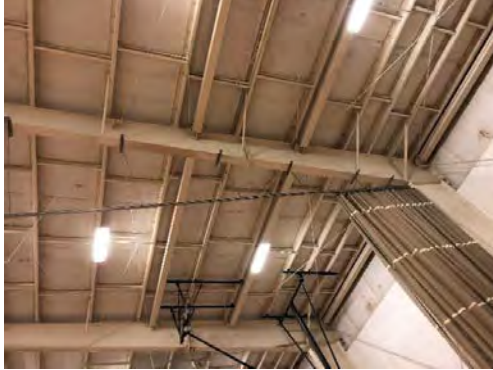
Photo 5.11: Moment frames, roof purlins and hanging partition wall support framing
