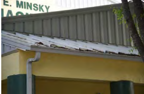
Photo 7.11: Lower front canopy roof.
