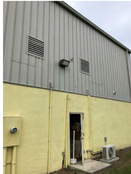
Photo: Gymnasium SE AHU – O/A Intake
