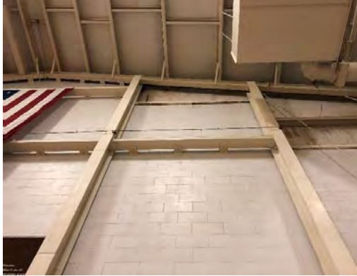
Photo 4.3: masonry walls to steel framing connection at the gym entrance elevation
