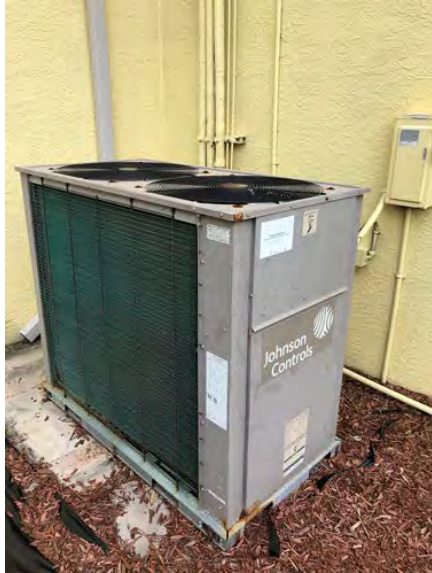
Photo: Gymnasium SE
