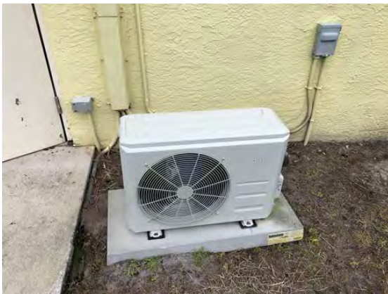
Photo: IT Room
