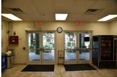
Photo 8.5: Storefront doors in good condition.
