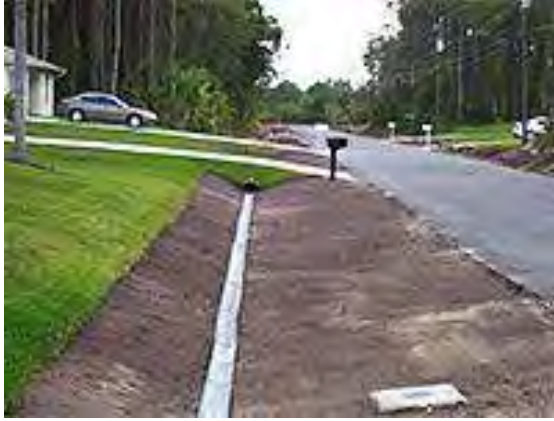
Image 3: Installation of a Standard Drainage Swale within PSL
