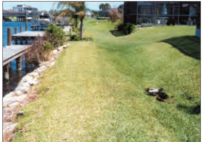
Figure 20. Leave a “Ring of Responsibility” to prevent pollution. Also note the swale and berm.
