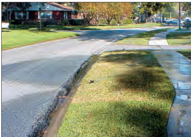
Figure 7. Poor design; sprinkler does not match area.
