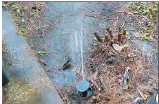
Figure 10. Object is interfering with spray pattern, resulting in poor distribution uniformity
