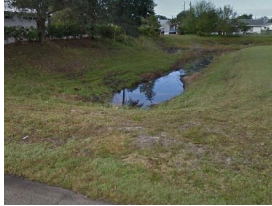
Evaluate and improve stormwater and drainage canal facilities
