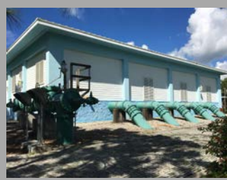
Booster pump station
